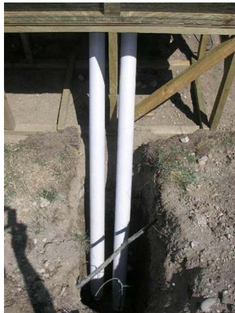
PVC pipes positioned under the cages and into a trench.
