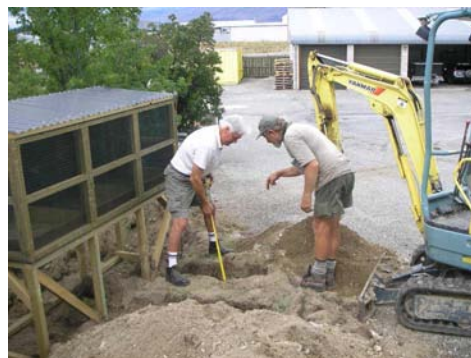
Tom Lamb (trustee) and Jonathan Rout (DOC) measuring the depth of the holes for the pipes.
