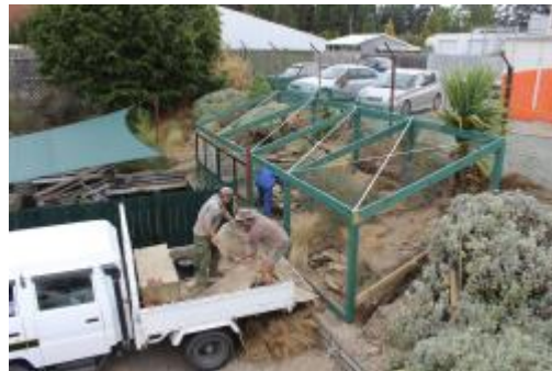
Constructing the new outdoor lizard enclosure
