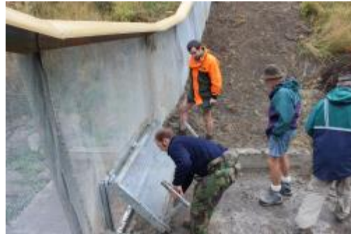
Inspecting a culvert.
