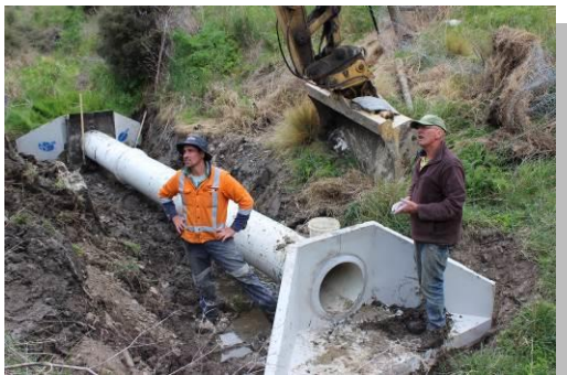
One of the culverts for the new fence.
